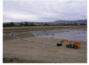
deployed. Once the geomembrane is properly placed, the material should be seamed as soon as practical. It is important to deploy the AquaMaster<sup>®</sup> material in a manner as to try and reduce the amount of field-seaming that will need to be completed.
