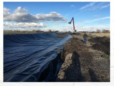
Cover soils should be dumped and leveled over the geomembrane and not pushed from one end to the other to minimize rolling and wrinkling of the geomembrane beneath the soils. Cover soil should always be placed from the bottom to the top of slopes to avoid stressing the
