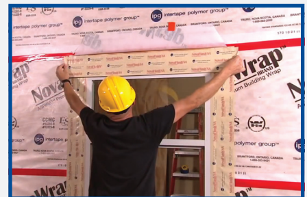
FIGURE 4: INSTALL HEAD FLASHING
