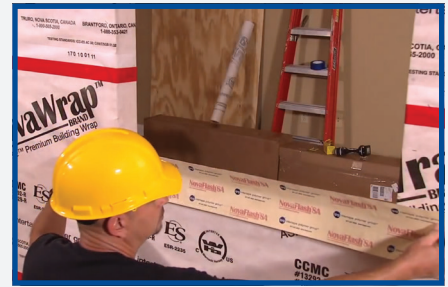
FIGURE 1: INSTALL SILL FLASHING
