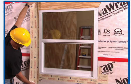
FIGURE 3: INSTALL JAMB FLASHING
