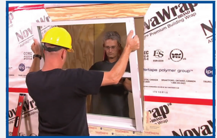
FIGURE 2: INSTALL WINDOW
