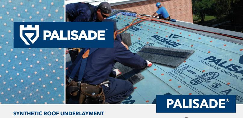
Palisade® synthetic roof underlayment is made from a completely waterproof multi-layer construction includes a top surface with Stronghold Skid Resistant Technology®, which is designed to provide roofers with superior walkability in the most demanding steep slope conditions of wet & dusty surface environments. It is lighter and 30x stronger than traditional asphalt felt products. Palisade is designed for use under metal, asphalt shingles, synthetic shingles, primed cedar shakes, slate and tiles.
